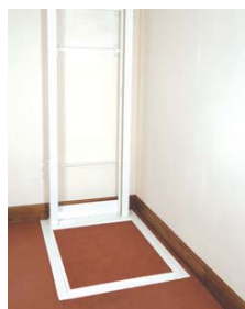
Upper room when lift downstairs
